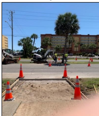
Forms for Concrete
