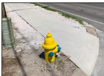
South Side Handicapped Ramp to the Beach Side Parking Area
