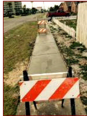
Fresh Cement Poured
